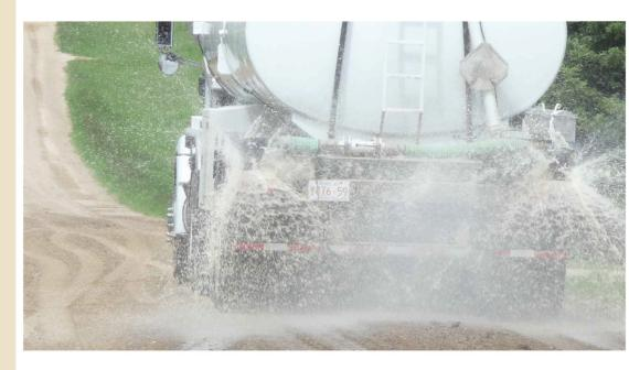
The municipality no longer uses oil as a suppressant since roads treated with oil are difficult to maintain and can become a hazard due to pot-holing.
