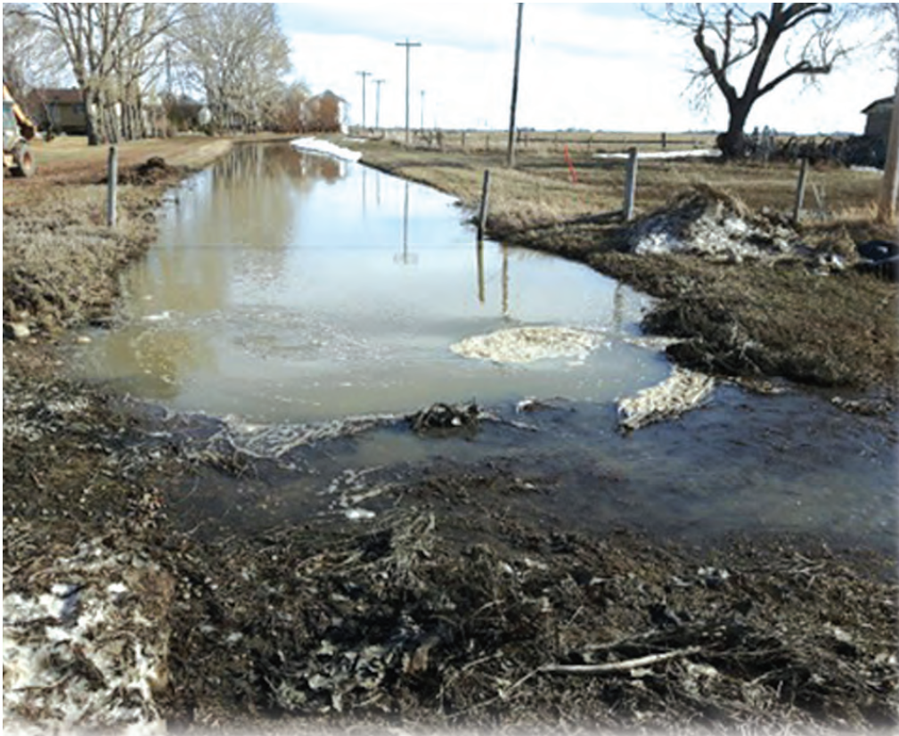
TID Lateral Overflowing at Highway Crossing Due to High Inflows, April 15, 2018
