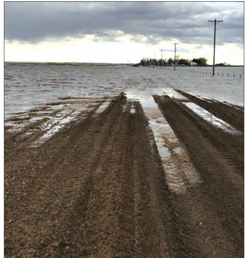
Intersection of highway 877 and Route 513, south of Grassy Lake
