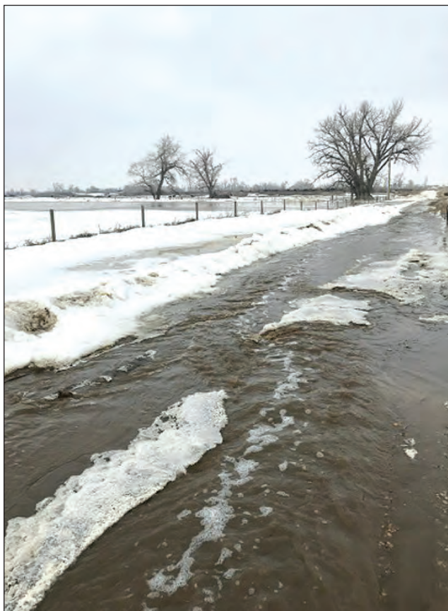
Range Road 17-2 North of Township Road 10-0 – Road Erosion
