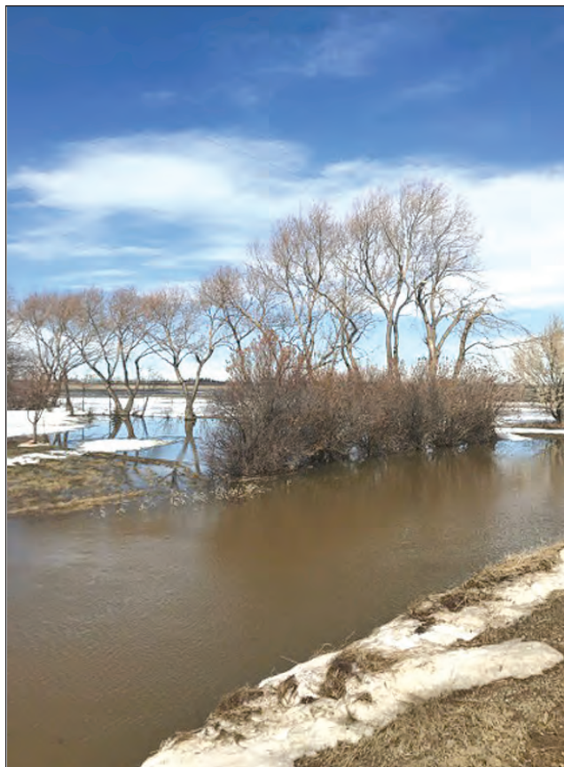
Range Road 16-2 between Township Road 9-4 and 10-0 – Cut approaches to save residences
