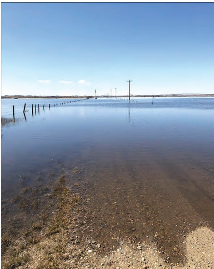
Range Road 18-3 – North of Enchant – Water covering 800m of Road
