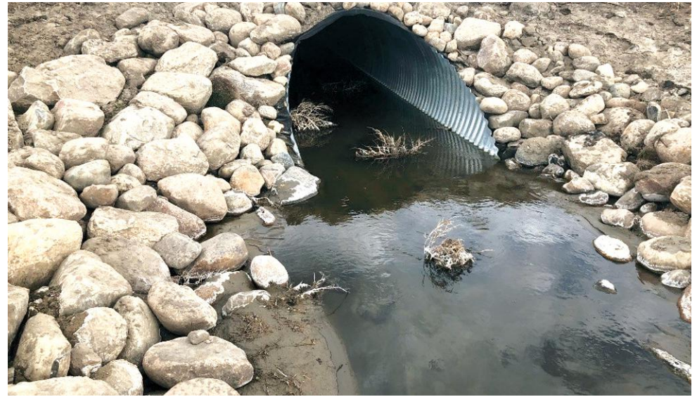
Bridge File 84230 – Completed upstream end
