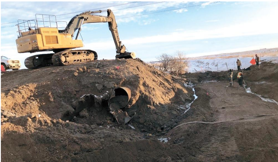
Bridge File 84230 – Excavation and base preparation
