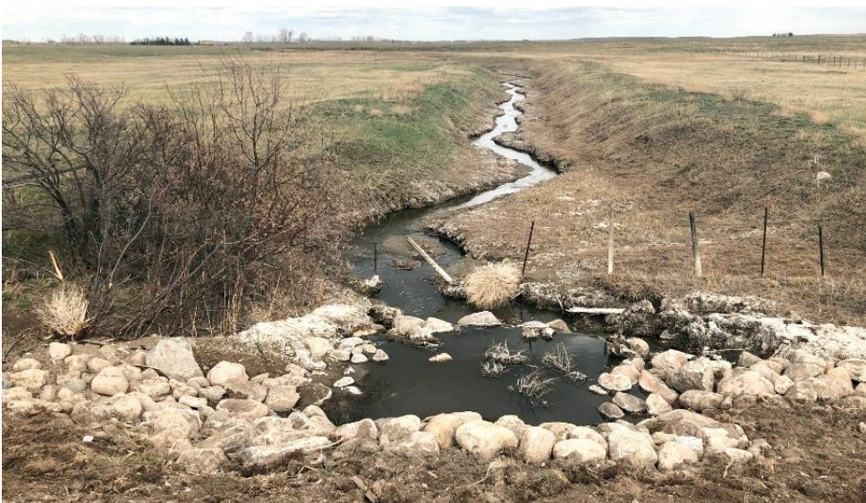
Bridge File 84230 – Completed downstream
