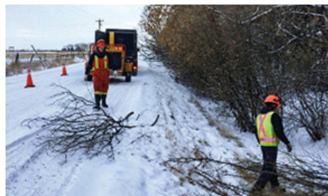
Crews clearing brush in the ditch.
