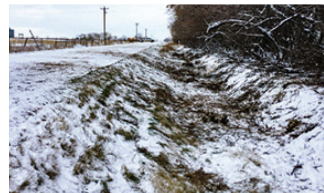
The same ditch after clearing.
