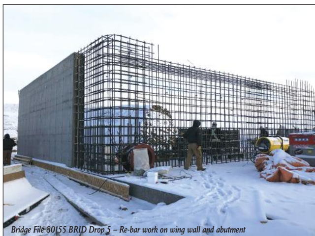
Bridge File 80155 BRID Drop 5 – Forming work on wing wall and abutment
