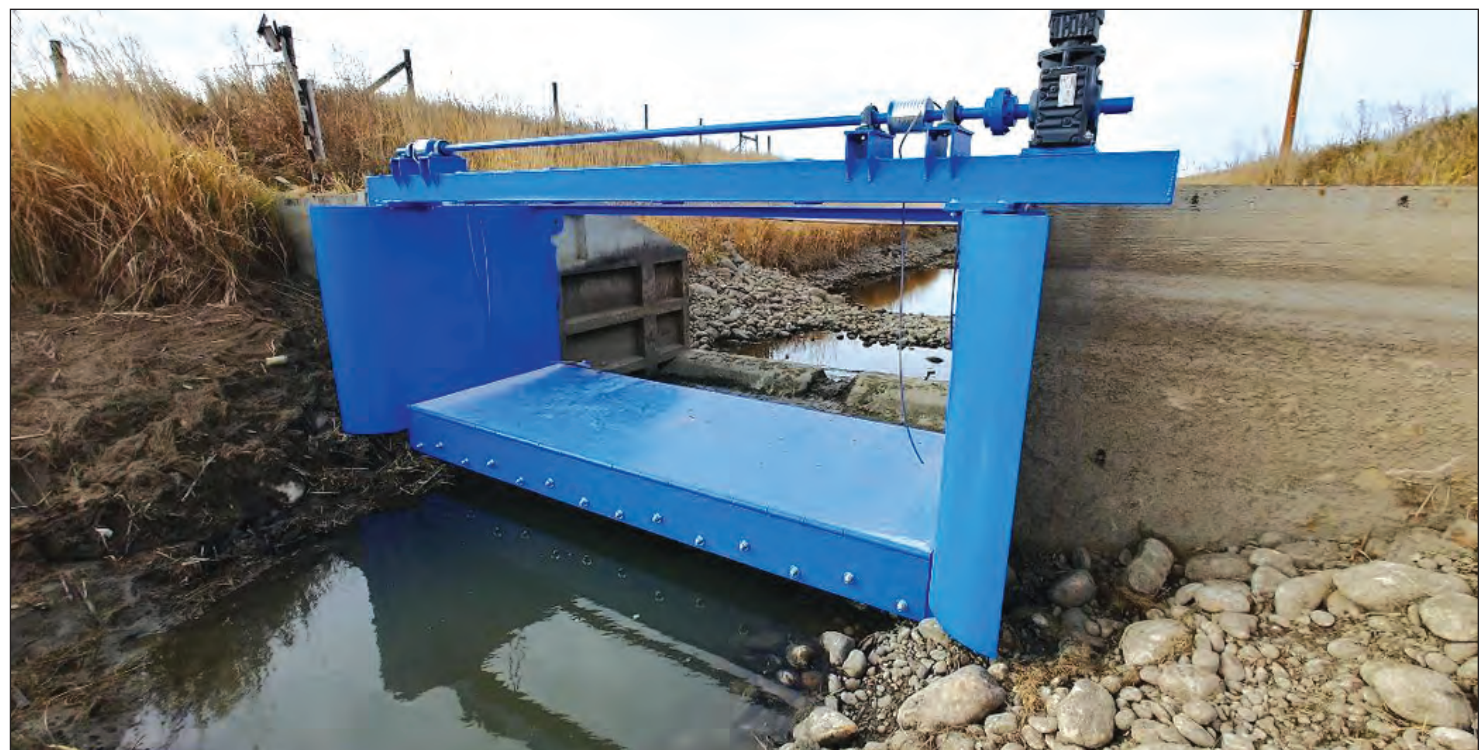
Lateral 2 East Horsefly Overshoot Gate Installed in November
